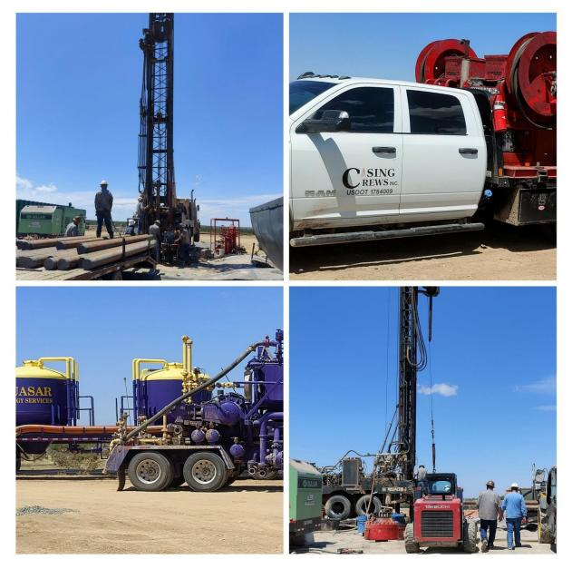
Blue Star Helium Limited | ASX:BNL | OTCQB:BSNLF 194 Hay Street, Subiaco, WA, 6008 ACN 009 230 835 | info@bluestarhelium.com | www.bluestarhelium.com The intermediate hole section of the well was drilled to approximately 1,110 feet and the hole has been cased and cemented. Shortly, a mandatory cement bond log (CBL) is to be run.
