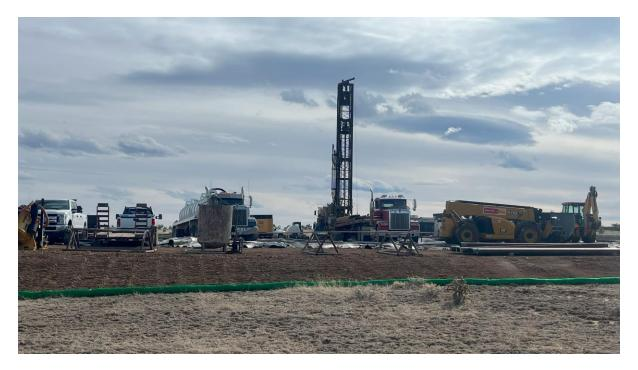
At TD wireline logging will then be conducted, followed by flow and pressure readings at the wellhead. This data will be used to estimate the production potential of the well based on the model built from existing data collected from the field as described below and public information available from the adjacent Red Rocks development.
