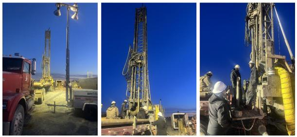
The photos above show drilling of intermediate hole section and driller Craig and CEO Trent Spry discussing the key casing point within the sealing formation above the targeted Lyons helium reservoir.
