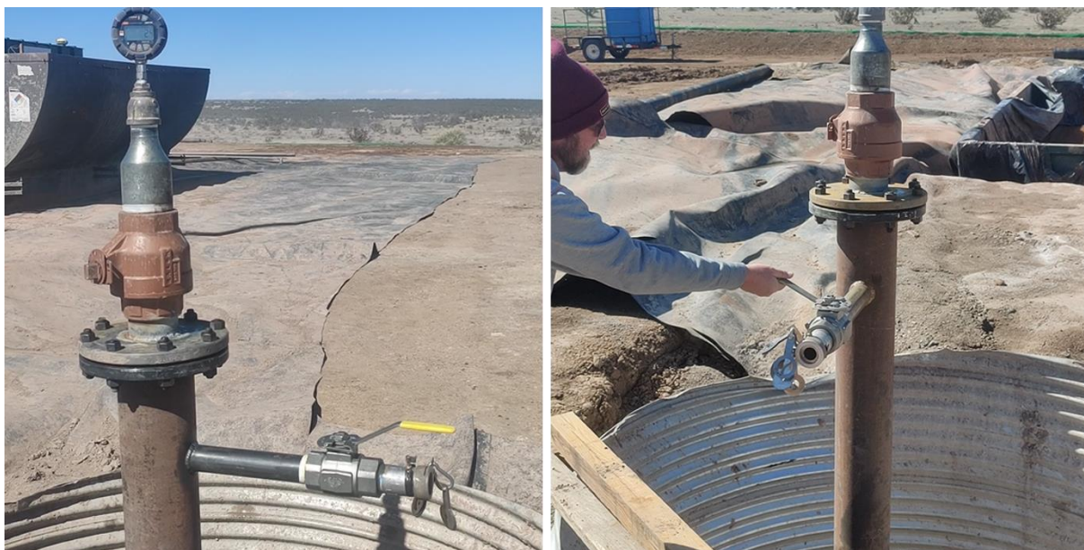
Well-head testing at Jackson 31 well, Galactica Project
